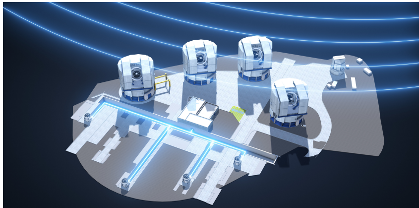
■ Figure 1 The instruments on Paranal, Chile. The four larger structures are the Unit Telescopes (UTs) housing various instruments. The four smaller structures are the movable Auxiliary Telescopes (ATs). The image shows light from each AT being directed through tunnels to the central VLTi laboratory, which is housed underneath the central building. Light may also be directed from the UTs to the central VLTi equipment. Credit: ESO/L. Calçada (eso.org).
