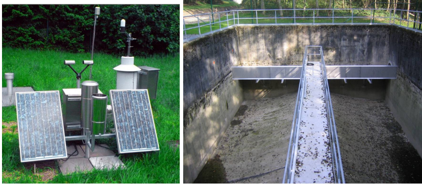
Fig. 1.13 Left: Rain gauge (pluviometer). Right: Stormwater tank.
